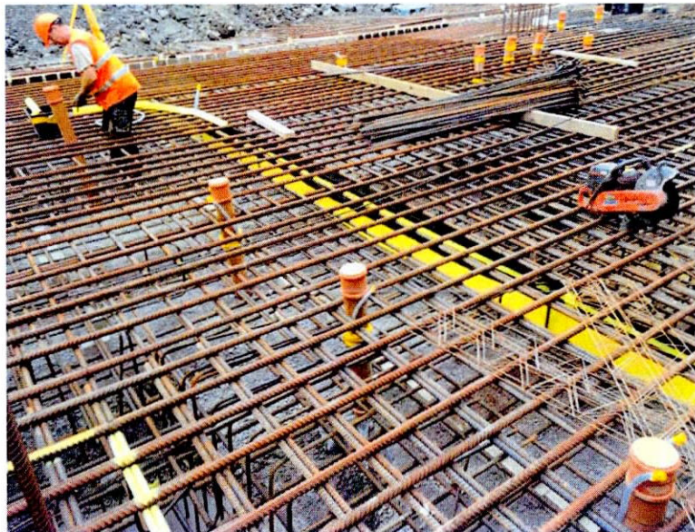
Photograph 3: Rascor White Tank Injection System in Basement Slab
