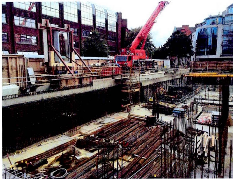
Photograph 1: Secant Piled Wall Supporting Perimeter Columns
